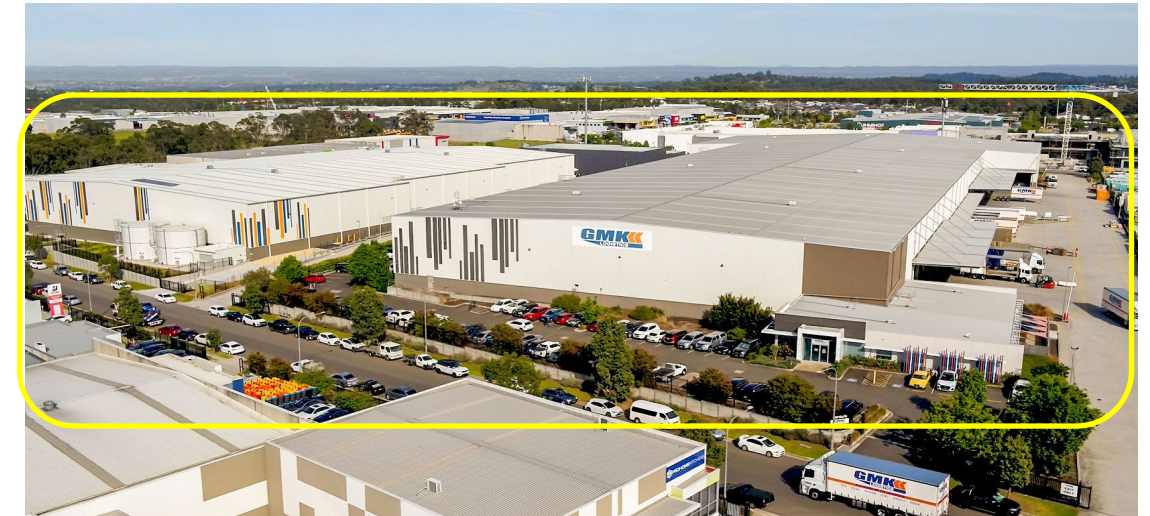
GMK Gregory Hills NSW (original on right, expansion on left)
