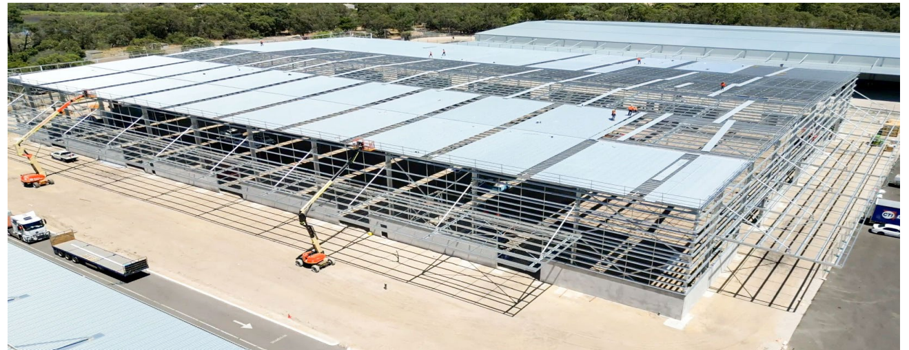
Development at 17 Lakes Road Hazelmere WA
